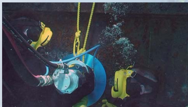
Navy Divers working to position the Underwater Friction Welding System to weld a stud in place.
